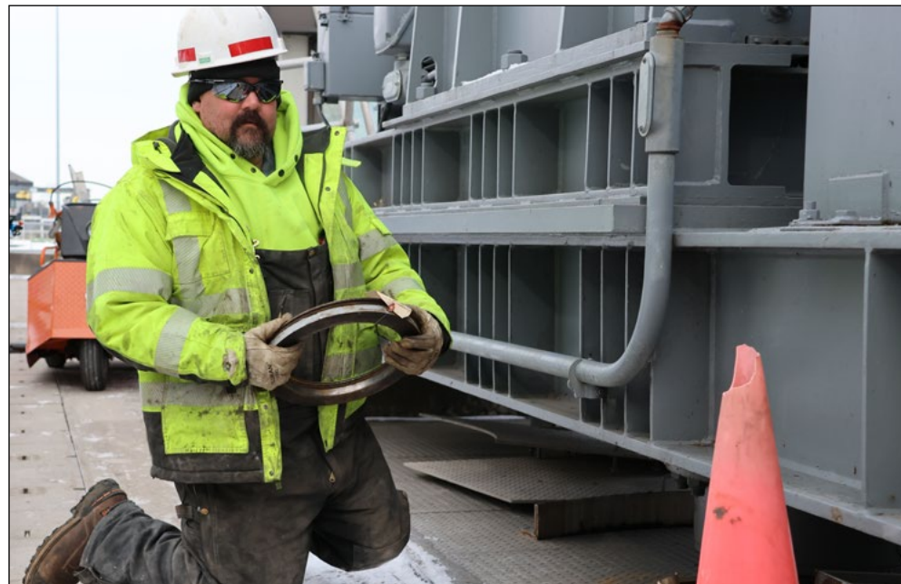
Noah Andow, maintenance and repair, getting a gudgeon pin shims cleaned and ready for installation at Lock and Dam 3, near Red Wing, Minnesota, Feb. 21. USACE St. Paul District photo by Elizabeth Stoeckmann
